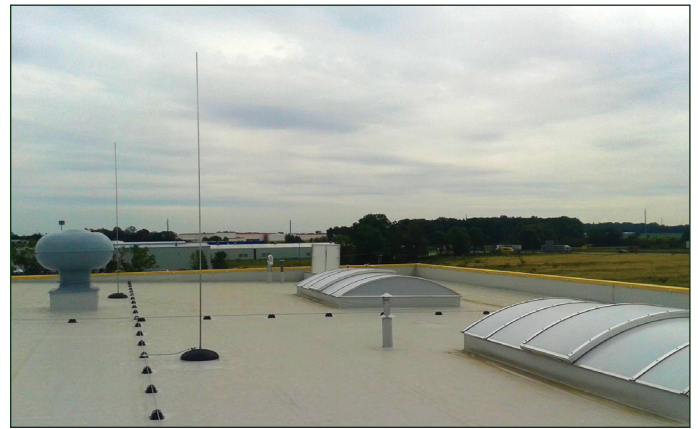
Figure AT:3 - Free-standing Air Terminals installed with 8mm diameter aluminium conductor
