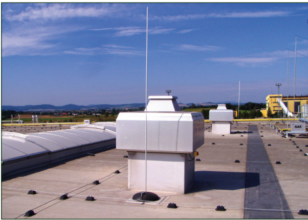
Figure AT:3 - Free-standing Air Terminals installed with 8mm diameter aluminium conductor
